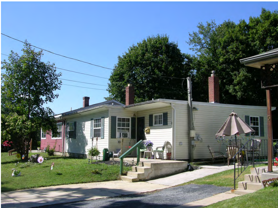
Photo 2: Plan B, north end (3) of 1-3 Foundry Street, Camera facing SW. Windows and siding replaced but prominent chimneys and flat roofline intact.
