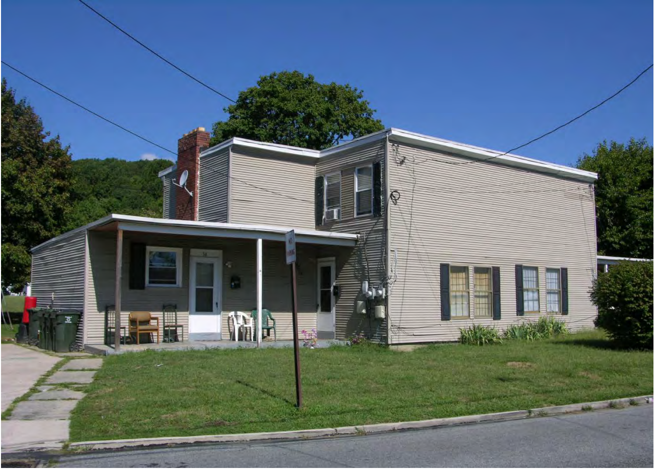
Photo 13: The most intact exterior of the A Plans (4-plex), 50-56 Foundry Street. Camera facing N.
