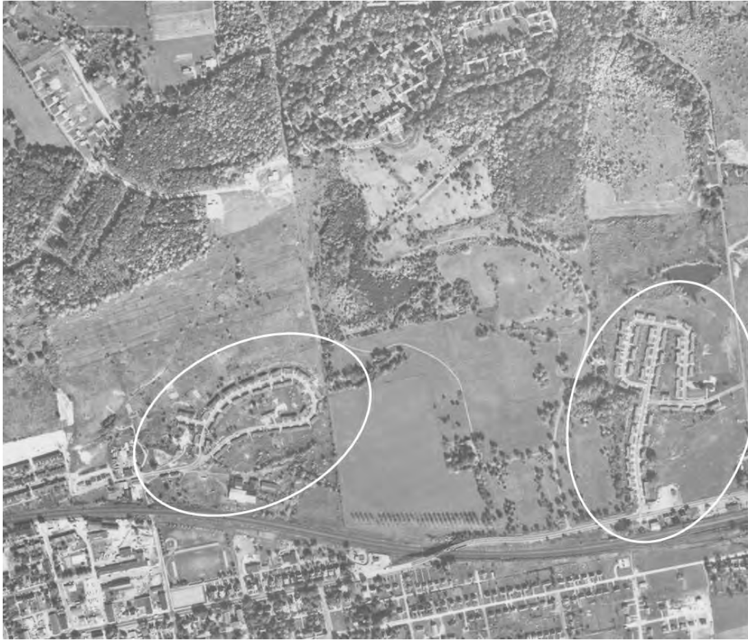
Figure 8: Historic aerial view, from pennpilot.psu.edu; photographed October 14, 1957; id# AHK-4R-69. Carver Court and Brandywine developments fully constructed.
