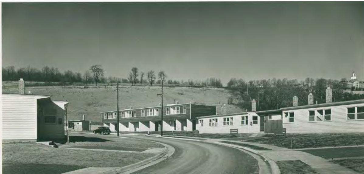
Figure 14: Standing in front of 89-91 Foundry Street, facing N. The Veterans Administration hospital is visible at the top of the hill to the right (east). The open hillside behind Carver Court later became heavily wooded. The Plan B house in the center of the photo may be the one destroyed by fire c.1970 (81-83 Foundry St.).
