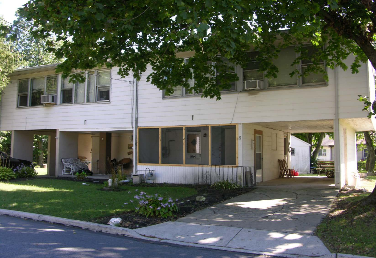
Photo 3: Plan C duplex, 2 and 4 Foundry Street. Camera facing E.
