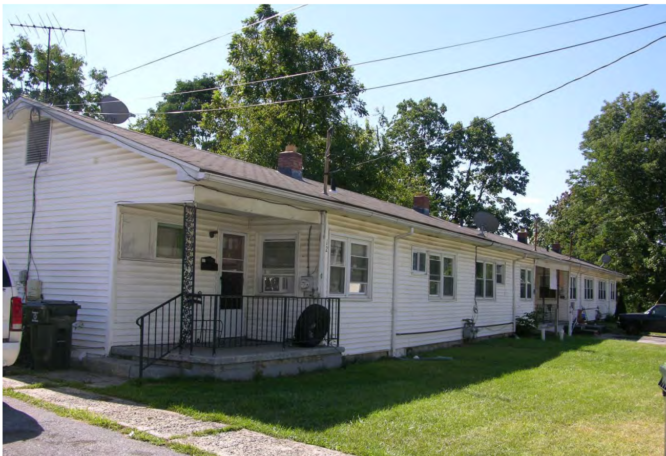
Photo 6: Row of Plan BB houses, with 12 Foundry in the foreground. Camera facing S.
