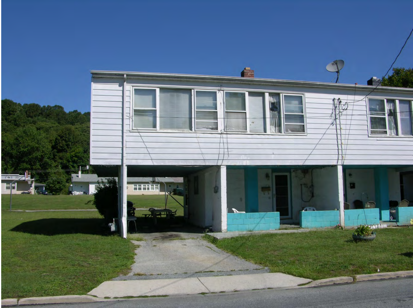
Photo 15: Detail of 64 Foundry St., end of a CC Plan, with basketball court visible in rear yard; rear open space was formerly part of Community Center, now associated with church property. Camera facing N.
