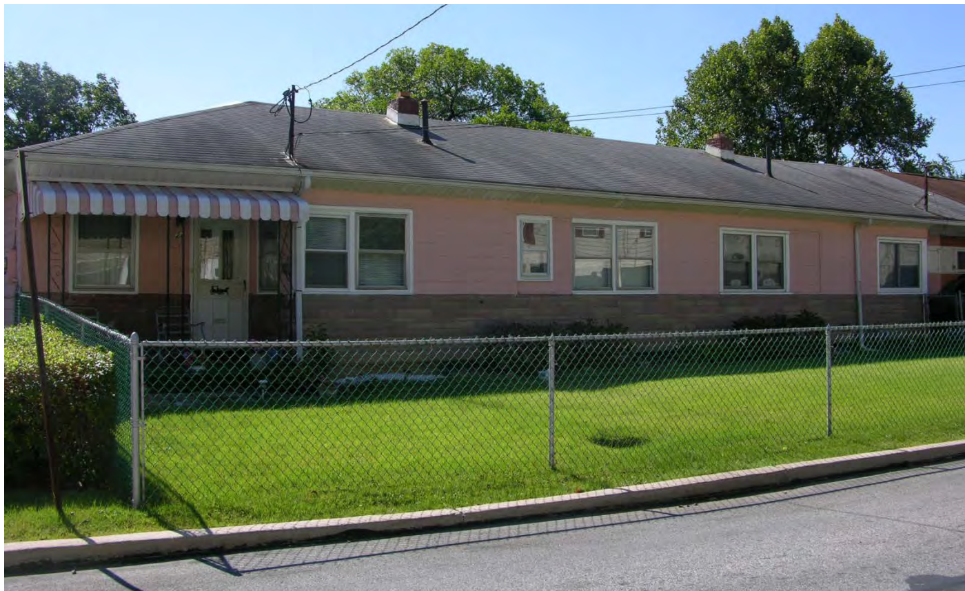
Photo 8: Houses 24 and 22 Foundry St. were combined into one residence. Half of a BB Plan. Camera facing SW.
