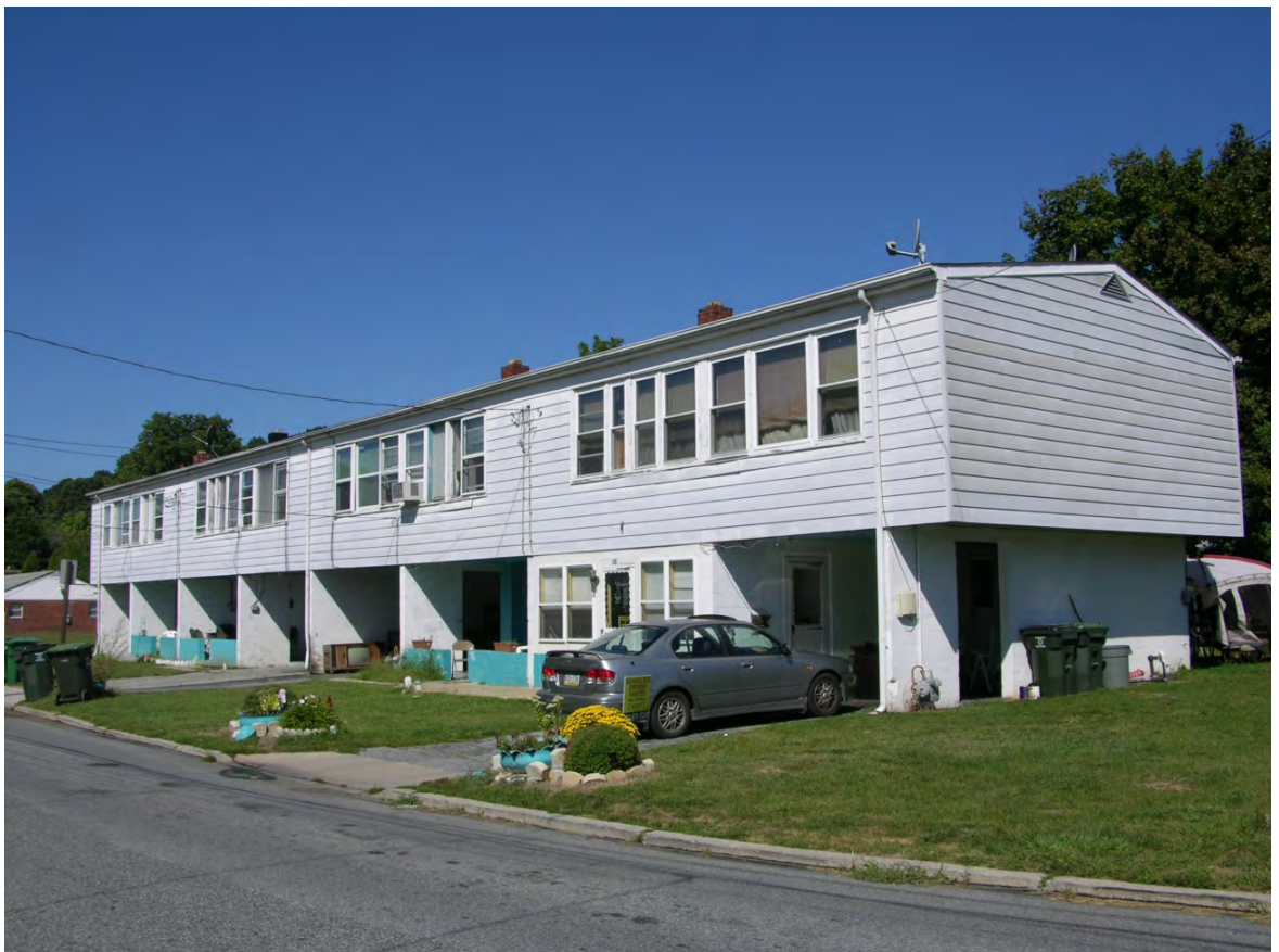
Photo 14: CC Plan 58-64 Foundry Street. One porch enclosed, all others and carports open. Camera facing W.
