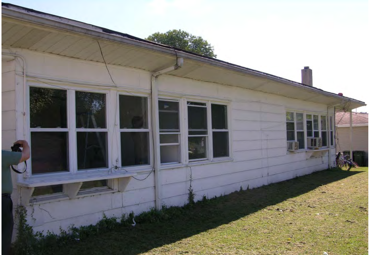
Photo 10: Rear elevation of 42 (left) and 44 Foundry Street, which retain original flower planter shelves with various size holes cut into shelf for pots. Original flat roof line. Plan B. Camera facing SE.
