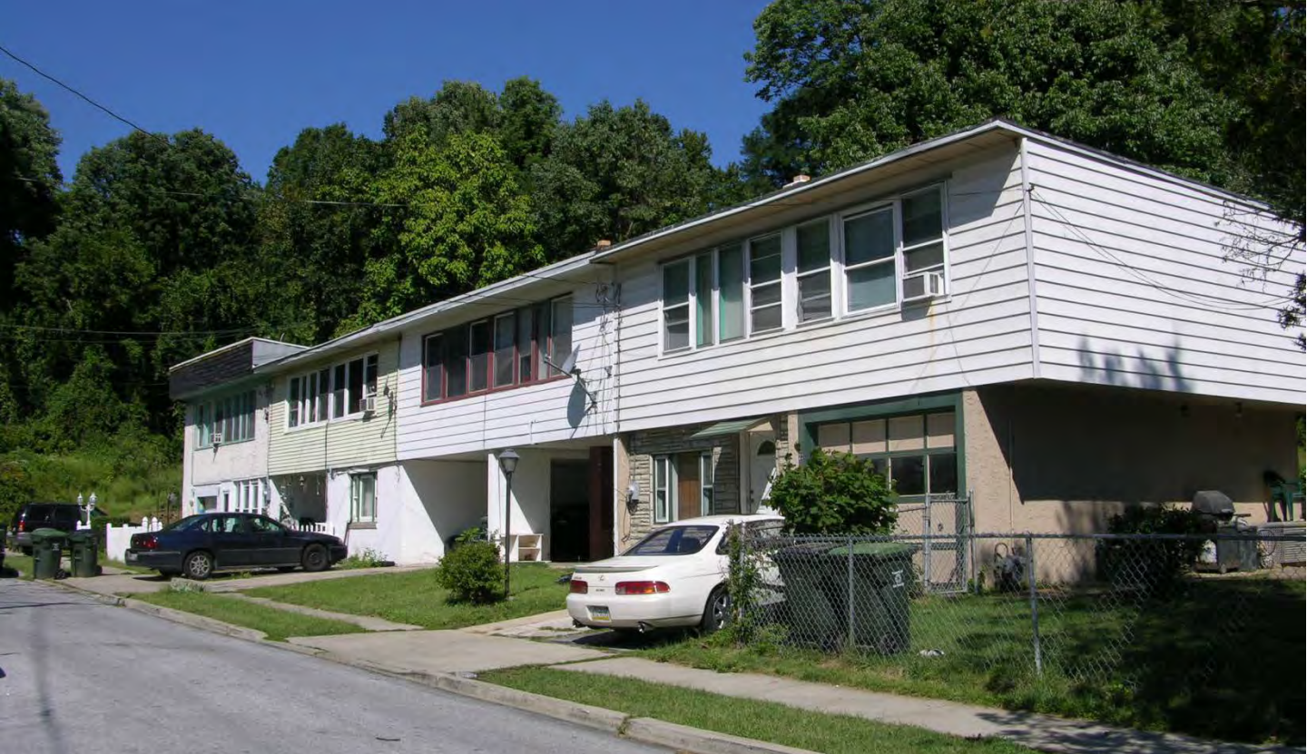
Photo 5: Houses on N side of Brook Lane; camera facing NW. Carport at E end has been enclosed as garage; some former porches enclosed. House at W end has a faux mansard roof. Plan CC.
